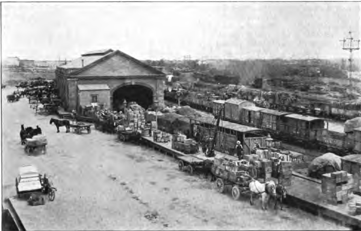
GOODS SHEDS, ADELAIDE RAILWAY STATION.
